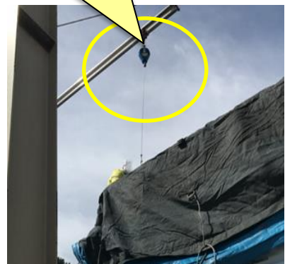
D-Shackle attached to cable clip
