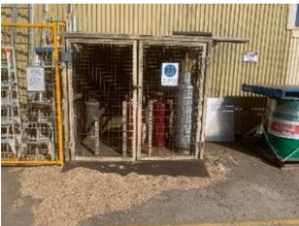
Gas bottles stored in caged area however signage needs to be updated and bottles were not all chained
