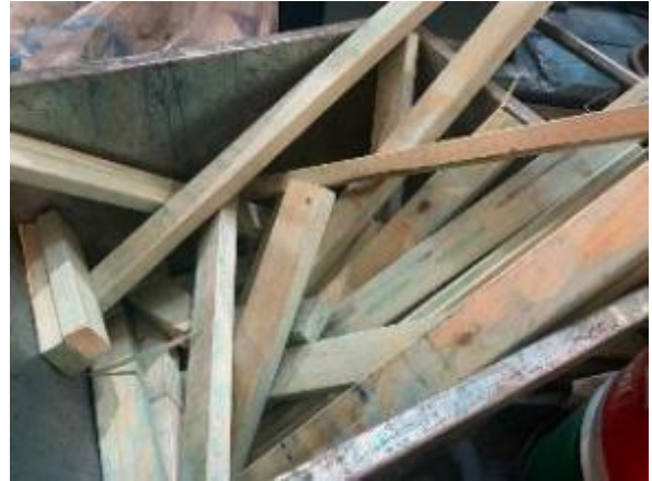
Waste management – as per the WMP – H2 treatment waste stored in bins that go to reuse at Borgs.
